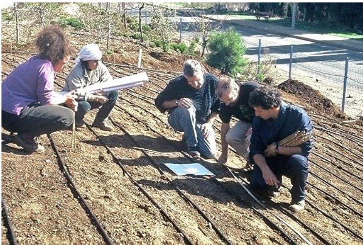
Volunteers laying irrigation pipes
